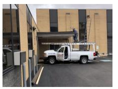
— A few weeks ago, Kenyon Roofing on Ohio River Boulevard was awarded the contract to Repair the Church Roof which included replacing blown away shingles, replacing worn shingles and securing lose shingles. They also sealed the loose gutters from leaking water. The roof over the garage and the porch area were attended to by securing the flashing and membrane against the wall. Water was coming through the basement area near
