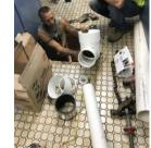
The rain water on the Catherine Street Roof side of the gym has now been diverted into the street; (2) A larger pipe was replaced in the school basement to keep the water from backing up through the existing water fountain onto the floor; and (3) a new
